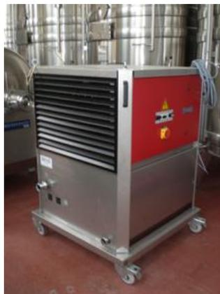
Figure 2.43: Portable packaged chiller unit
