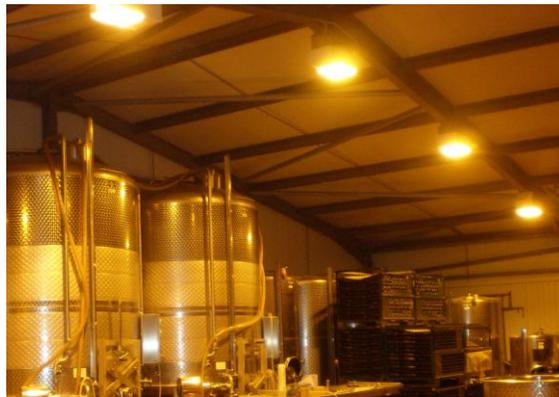
**Figure 2.58:** High pressure sodium fittings used in a general tank area
