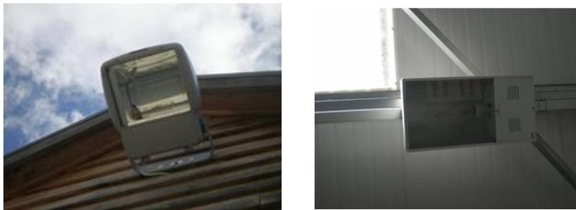
**Figure 2.56:** External security fitting with a metal halide lamp (left) and high bay metal halide HID fitting used in a production area (right)
