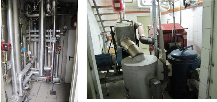
**Figure 2.72:** A 10kWc NH<sub>3</sub>/H<sub>2</sub>O absorption refrigeration unit (left) and 50 kWth wood chip furnace connected to a 3 kWel Stirling engine (right)
