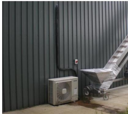
Figure 2.40: External spilt condenser/fan unit for AC
