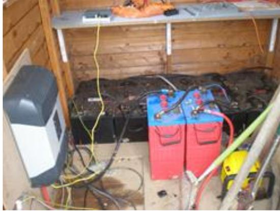
**Figure 2.15:** PV system inverter with battery storage
