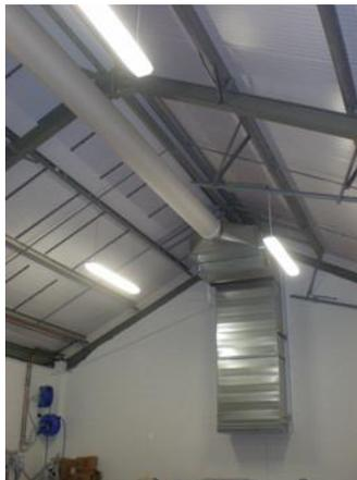
**Figure 2.36:** A fabric forced-air ducted AC installation
