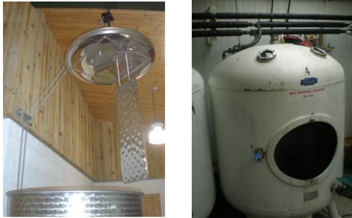
**Figure 2.47:** Water cooled tanks; lid mounted heat exchanger (left) and tank mounted heat exchanger (right)
