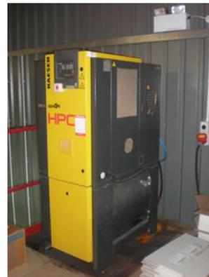
**Figure 2.64:** Older air compressor unit located outside in dedicated lean-to shelter (left) and internal packaged air compressor unit, complete with integrated dryer (right)
