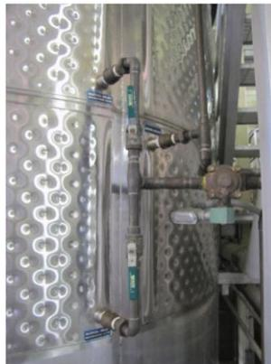
Figure 2.46: Fixed glycol cooling connection to tank heat exchanger
