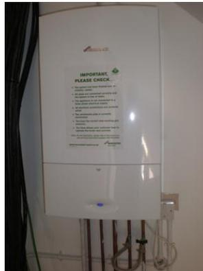
Figure 2.66: Gas condensing, combination boiler used in an English winery
