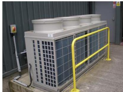
Figure 2.41: External packaged chiller unit (vertical air discharge) for process cooling
