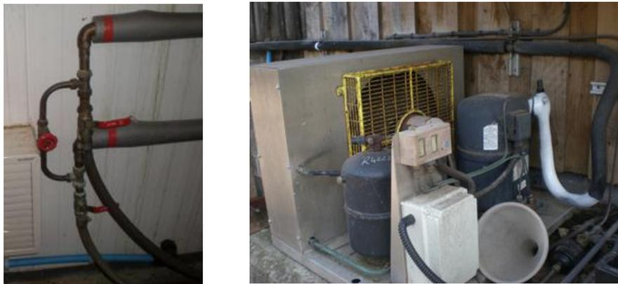
Figure 2.50: Missing or poor insulation on refrigeration pipework
