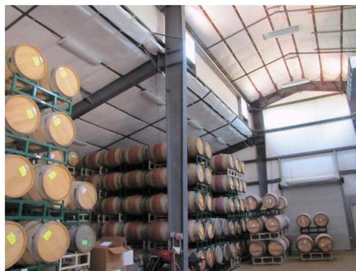
**Figure 2.31:** Good use of structural retro-fit insulation in a barrel room store
