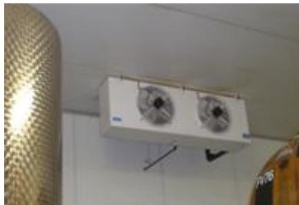
Figure 2.45: Fan coil unit
