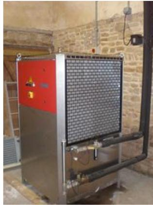
Figure 2.42: Fixed packaged chiller unit located indoors
