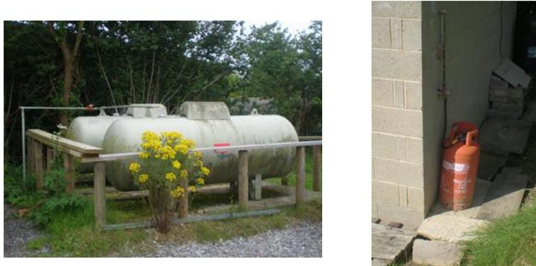
Figure 2.9: Examples of gas fuel storage/supply
