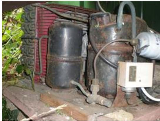
Figure 2.49: Old, inefficient refrigeration plant
