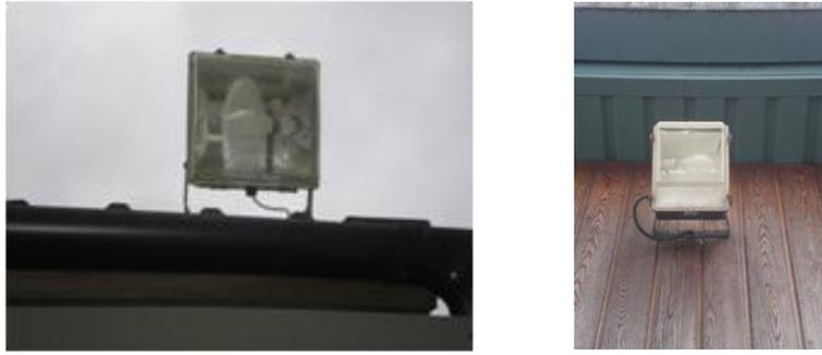
**Figure 2.57:** External high pressure sodium fittings
