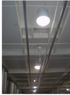
**Figure 2.62:** External and internal images of the daylighting system in the Pinot Noir facility in a Californian winery
