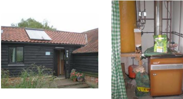
**Figure 2.16:** Example of a roof mounted solar thermal installation and integral bio-mass burner/boiler
