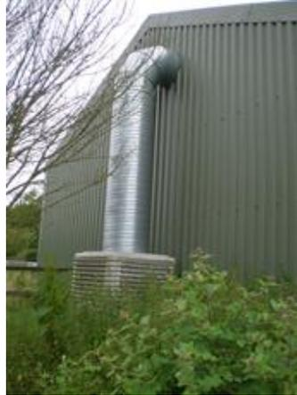
**Figure 2.37:** A ducted evaporative (swamp) cooler
