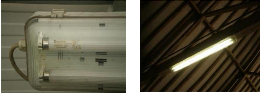
**Figure 2.55:** T-8 (left) and T-5 (right) fluorescent lamp fittings in English wineries
