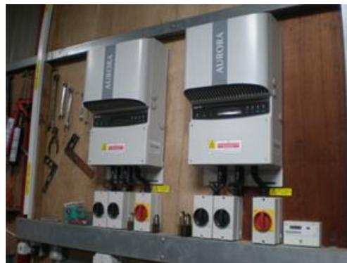
**Figure 2.14:** PV system inverters (direct building grid supply)
